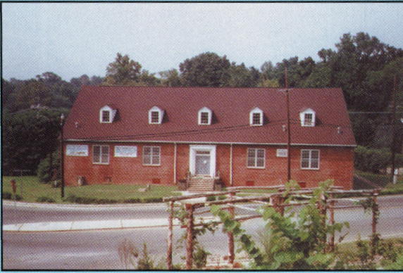
Figure 5. The Sazapahaw Community Center, Built by B. Everett Jordan and the Sellers Manufacturing Company. Privately funded, it houses a wide range of community athletic and social activities.
