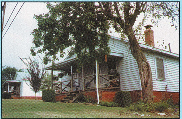
Figure 4. Former Saxapahaw mill houses now serving as rentals, neatly landscaped and maintained.
