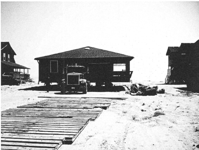
Figure 2. The movement of a house away from the ocean side of a barrier island to protect it from erosion and storm surge damage, Nags Head, North Carolina.
