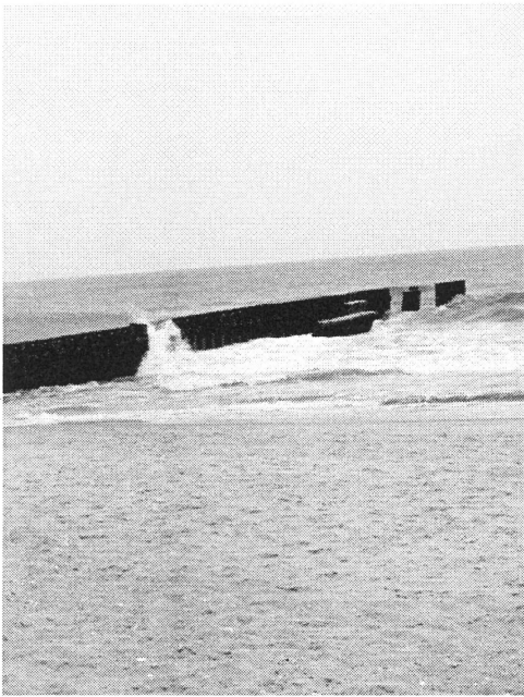
Figure 3. Left: Groin used to protect the Cape Hatteras Lighthouse before it was moved. Such hard structures are usually only permitted in North Carolina to preserve sites of historical significance or navigational importance. Right: Sand bags or tubes used to protect a house in Rodanthe, North Carolina. Soft structures are occasionally permitted to protect residential property (Photos: D.W. Gamble).
