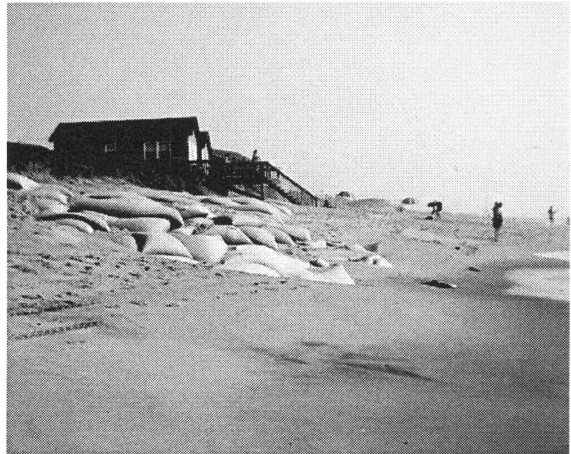
Figure 3. Left: Groin used to protect the Cape Hatteras Lighthouse before it was moved. Such hard structures are usually only permitted in North Carolina to preserve sites of historical significance or navigational importance. Right: Sand bags or tubes used to protect a house in Rodanthe, North Carolina. Soft structures are occasionally permitted to protect residential property (Photos: D.W. Gamble).
