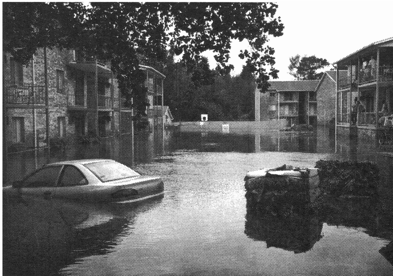
Flood waters at the apartments shown in the photo above. Notice the students on their balconies looking over the destruction. On the right are two tobacco bails that floated in from a warehouse upstream (photo by Bill Edwards).
