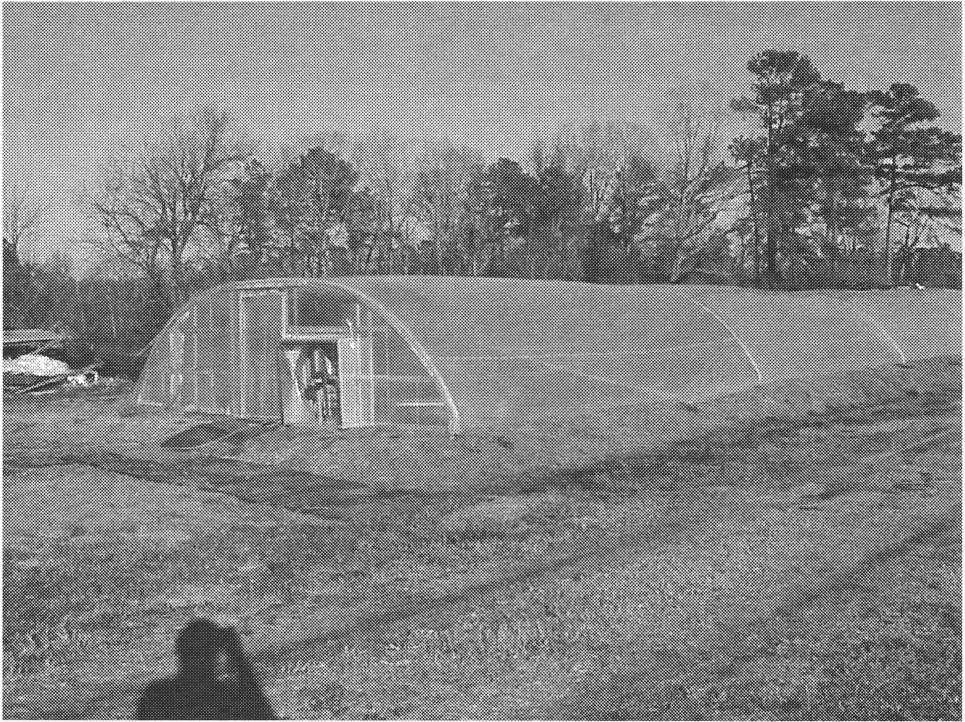
Figure 1. Greene County, North Carolina duckweed greenhouse showing inflated plastic covering and excavated earthen tank.
