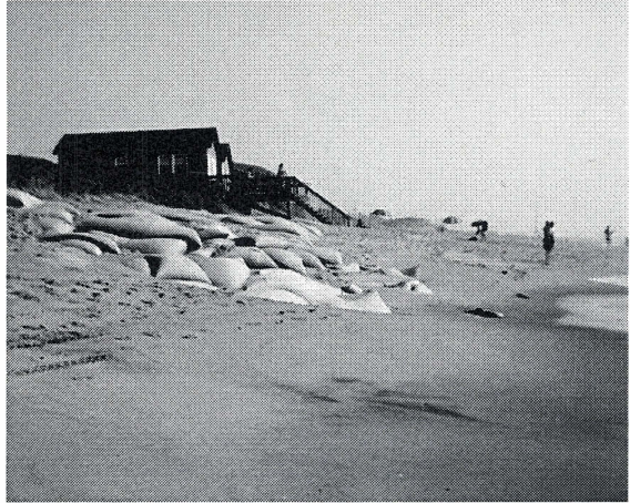
Figure 3. Left: Groin used to protect the Cape Hatteras Lighthouse before it was moved. Such hard structures are usually only permitted in North Carolina to preserve sites of historical significance or navigational importance. Right: Sand bags or tubes used to protect a house in Rodanthe, North Carolina. Soft structures are occasionally permitted to protect residential property (Photos: D.W. Gamble).
